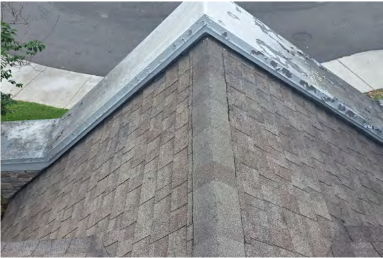
Remove and replace wall coping #2
