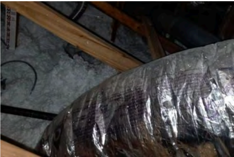
Existing attic insulation
