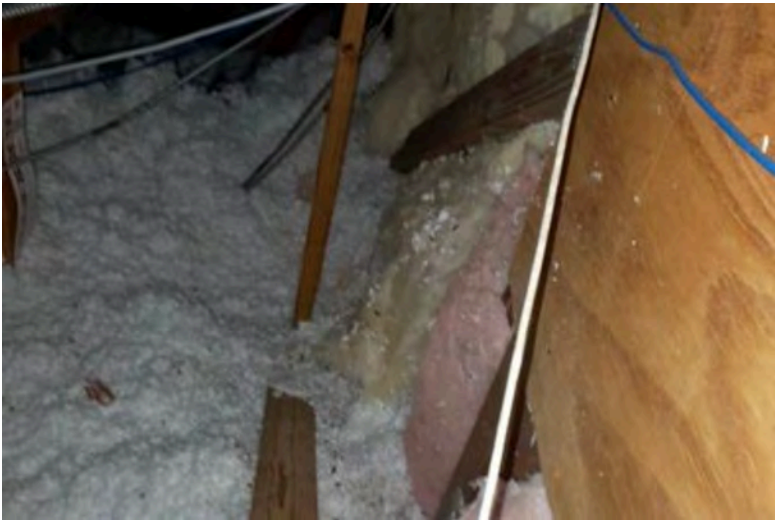
Existing attic insulation #2
